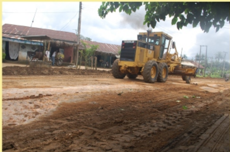
Grading Works in Abak 10 Abak L.G.A. Akwa Ibom State.
